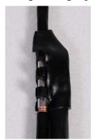
5 Use the remainder of the self-amalgamating tape to wrap the complete assembly. Press the tape edges together so that there are no gaps.
