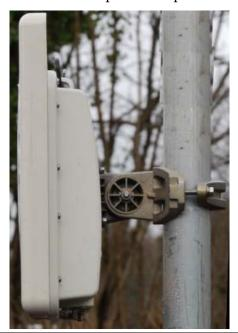
If LPU mounting option 2 (U-bolt) has been chosen, mount the LPU using the U-bolt bracket. The LPU must be vertical with cable glands facing downwards.
