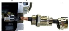
Support the drop cable and gently hand screw the gland body into the unit until the O ring seal is flush to the unit body.
