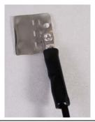
Fold the ground wire strap around the drop cable screen. Fit cable ties and tighten with pliers.
