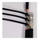
Cut the surplus from the cable ties. Cut a 38mm (1.5 inches) section of self-amalgamating tape and fit to the ground cable lug. Wrap the self-amalgamating tape completely around the lug and cable.
