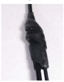
Wrap a layer of PVC tape, starting from 25mm (1 inch) above the outer jacket and finishing 25mm (1 inch) below the self-amalgamating tape, over lapping at half width.
