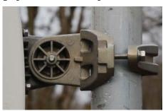
Adjust the elevation and azimuth of the unit to achieve an approximate visual alignment (does not apply to connectorized ODUs). Tighten both nuts to the required torque settings of 14 Nm (11 lb ft).
