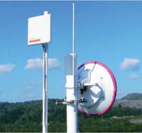
Gas utility connectivity, Siberia
