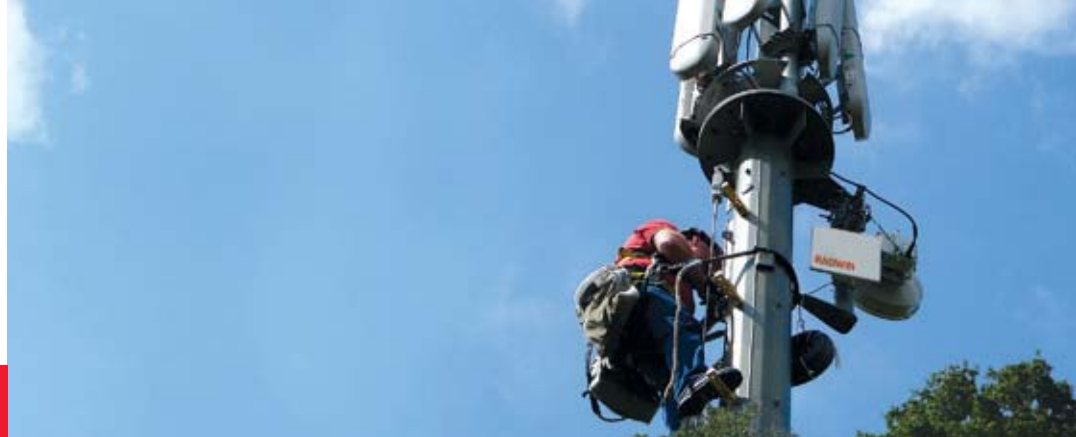
Cellular backhaul installation, USA
