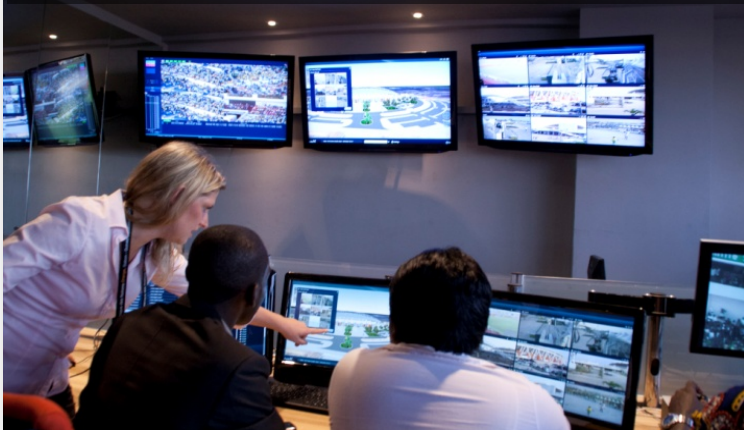
Real Time Video Monitoring at Control Center
