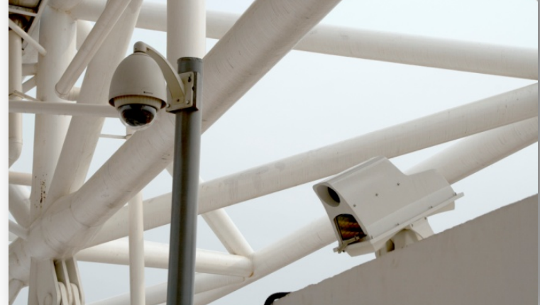
High Capacity connectivity to Stadium Cameras
