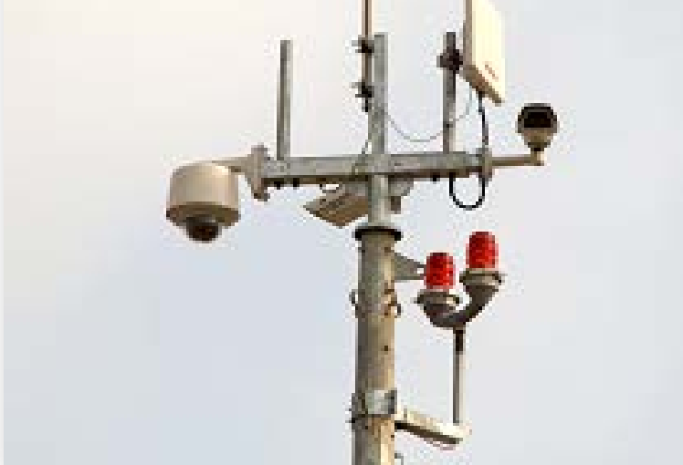
4 Cameras (3 Fixed, 1 PTZ) – 12Mbps by HSU 520
