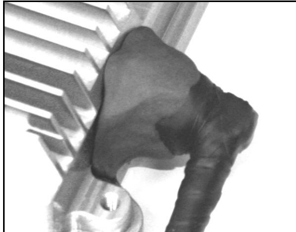
Figure 21: Weatherproofing - RF Cable Pt-4
