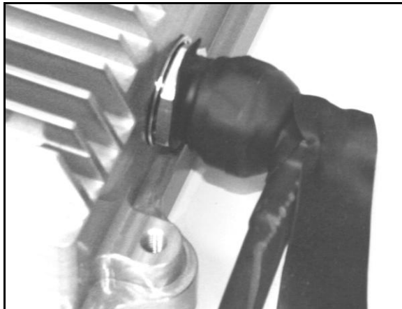
Figure 19: Weatherproofing - RF Cable Pt-2
